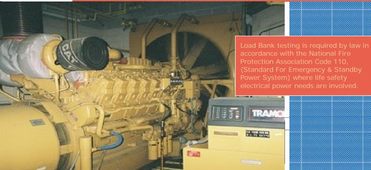
Load Bank Testing confirms the ability of your generator to produce a given kW and attain proper engine operating temperature.
